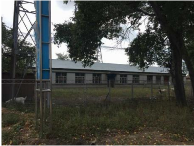
Figure 1. Civil relic buildings before renovation
